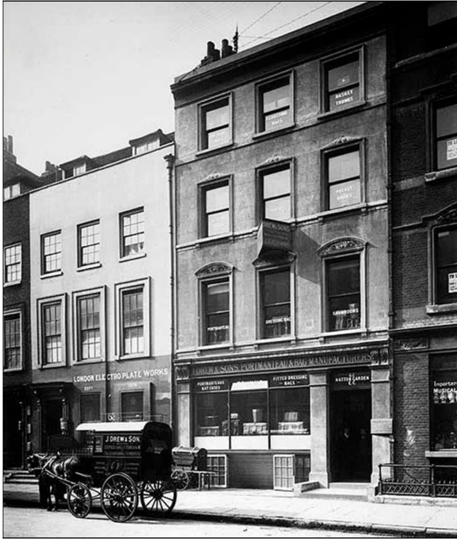
Hatton Garden, London's principal diamond and jewellery quarter, in the 1920's — a key setting of the novel
